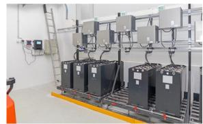
**OSHA Standard 1926.441(b)(1)** Battery charging installations shall be located in areas designated for that purpose.
