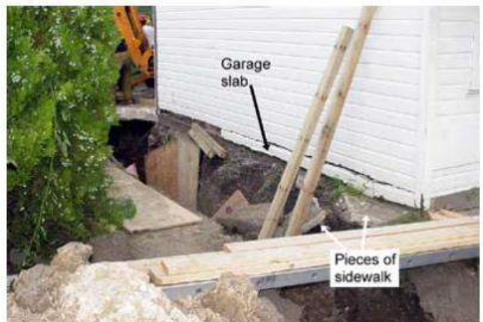
Two views of the scene of a fatal trench cave-in. Notice there is no protection in place to avoid cave-in hazards.
