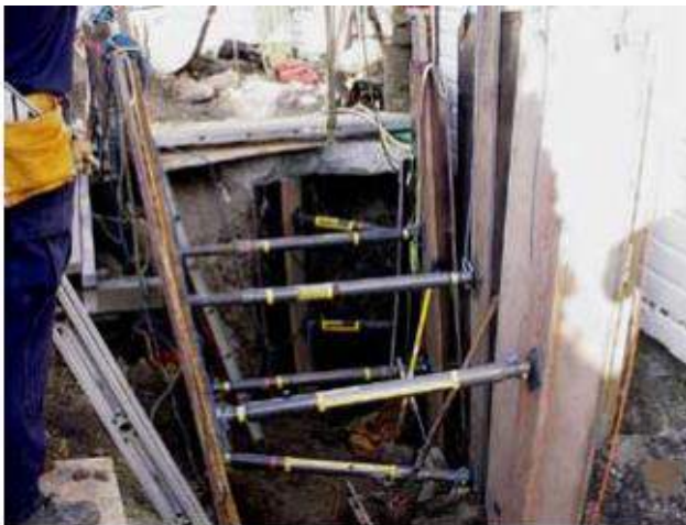
Scene of a fatal trench cave-in after cave-in protection was installed to safely remove the deceased worker.
